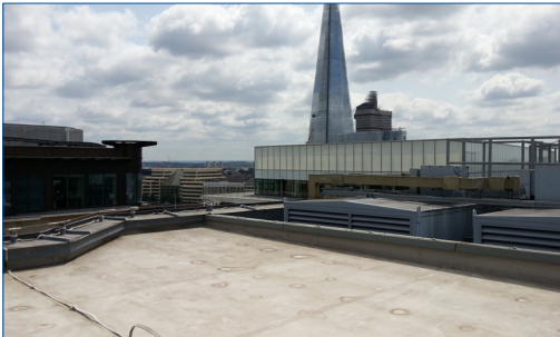
Roof cleaned and prepared
