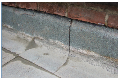
Leaking joints
